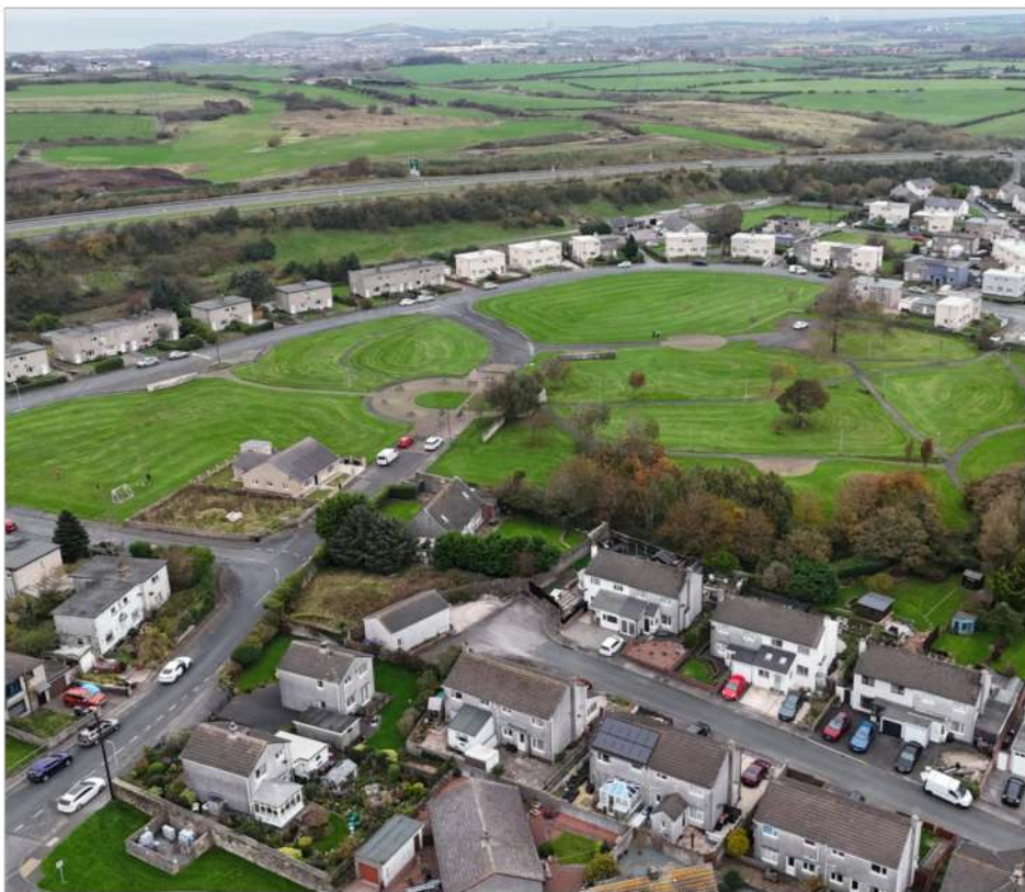
Arial View of Site from South East
