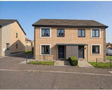
Elevation Material - Window Surround
